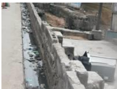
Drainage at Gbenla blocked by waste and collapsed portion of drainage structure
