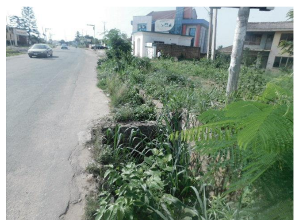
Plates 1.11 to 1.12: Drain blocked by silt and vegetation along Awolowo Road, Bodija.
