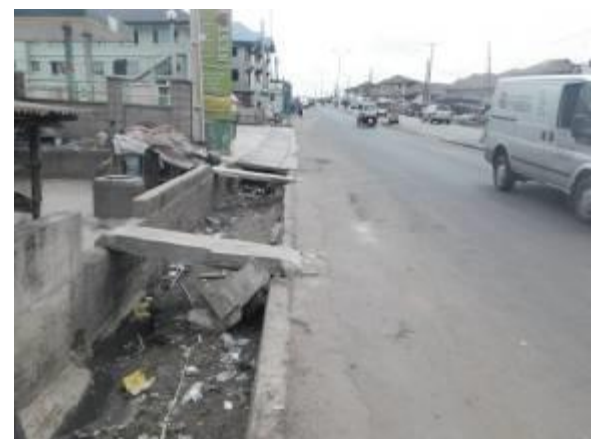
Plates 1.7 to 1.8: Collapsed portion of drain and blockages at Gbenla, Oje
