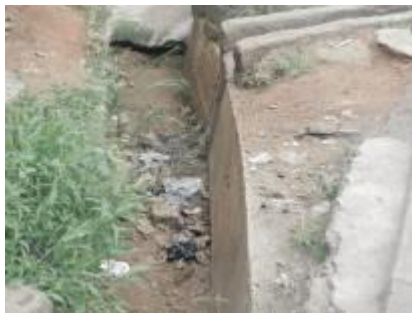
Blocked drainage along Total Garden to Adeoyo Road.
