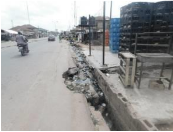
Plates 1.7 to 1.8: Collapsed portion of drain and blockages at Gbenla, Oje
