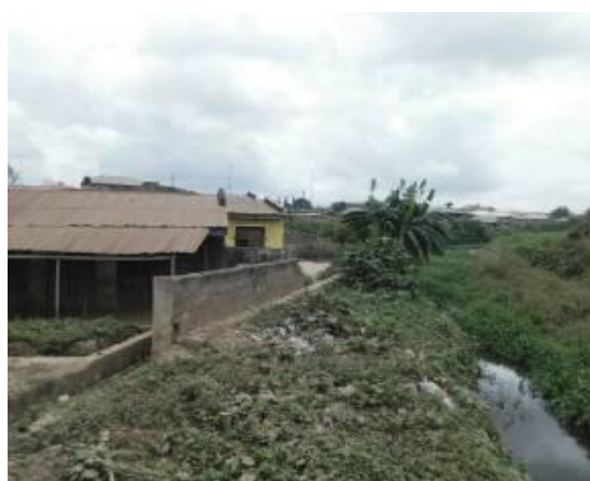
Plates 1.1 to 1.2: Onilu channel blocked by vegetation and solid waste,
