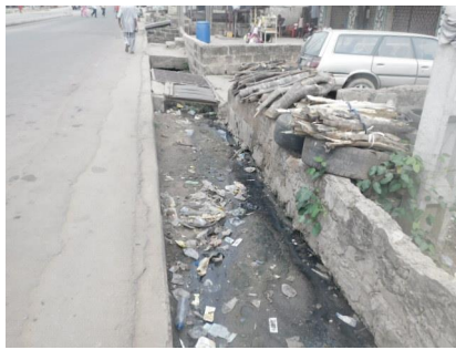
Drainage at Gbenla blocked by waste and collapsed portion of drainage structure
