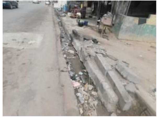
Plates 1.7 to 1.8: Collapsed portion of drain and blockages at Gbenla, Oje
