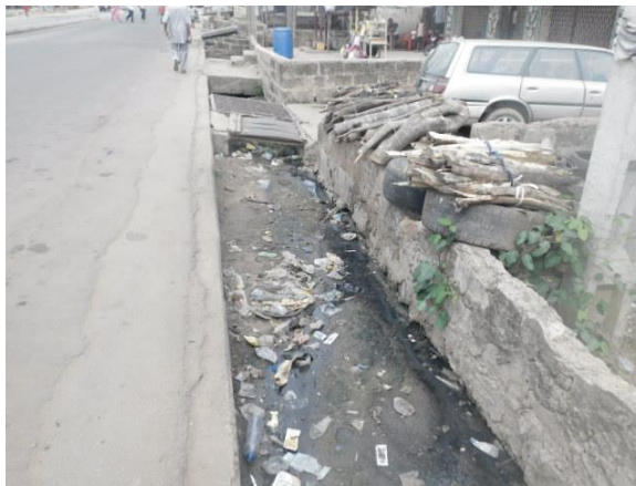
Plates 1.8 to 1.10: Silted and blocked drainage at Temidire, Oje
