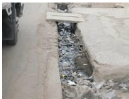
Blocked drainage around UCH
