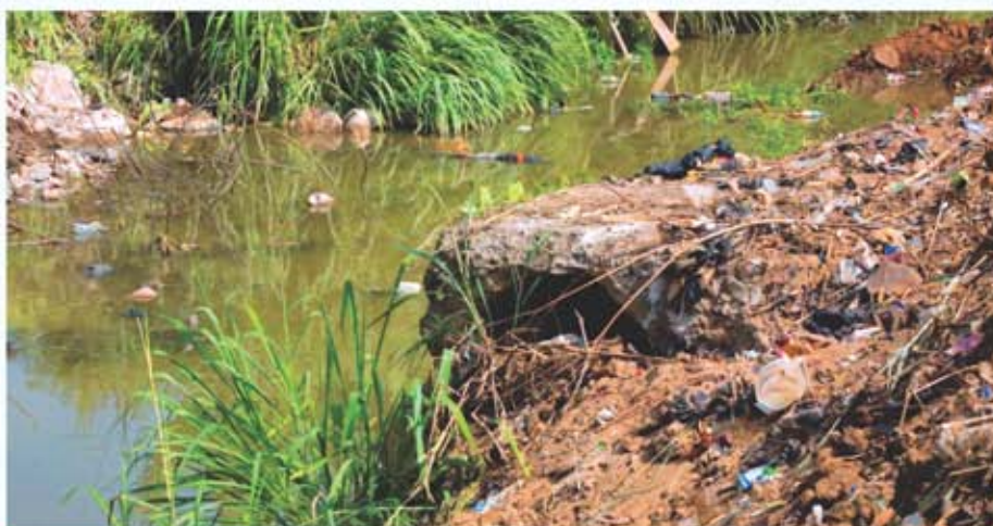
The collapsed Francis Okediji culvert at Old Bodija Area pre-intervention
