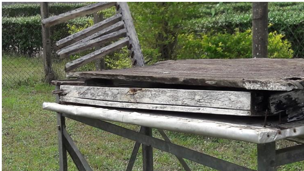
Plate 14: Status of Stevenson screen at Observatory site of CRIN in Ibadan
