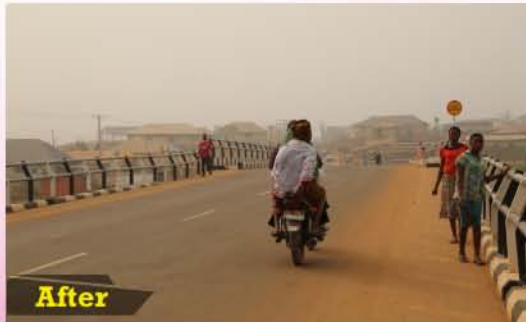
Construction of 2-span Bridge of 15m each at Ogbere Pegba with approach road and side drain.
