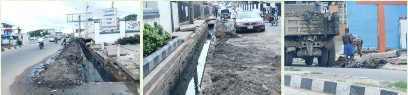
Pictures of drainage clearing, where excavated materials were promptly evacuated
